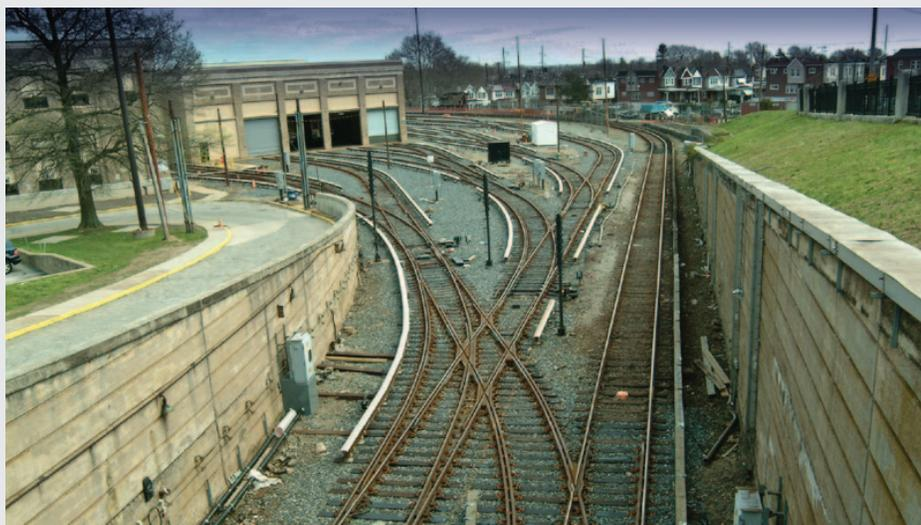
As part of SEPTA's Fern Rock Yard Renewal Project in Philadelphia, Pa., RailWorks Track Systems rehabilitated the tracks and turnouts leading to the entrance of the South yard and car repair facility. The crew removed old track, excavated, constructed new track and installed contact rail and coverboard. Similar work was performed in the North yard.
