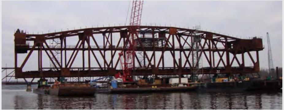
For several weeks, RailWorks crews boated daily to their worksite-on-barges to build track for a new lift span for the Burlington Bridge near Burlington, Iowa. BNSF Railway operates the track on the bridge extending across the Mississippi River.
