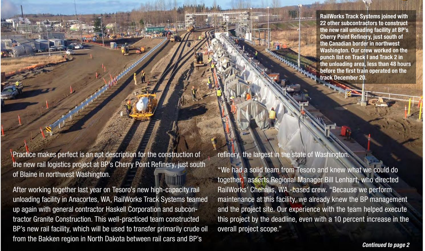
RailWorks Track Systems joined with 22 other subcontractors to construct the new rail unloading facility at BP's Cherry Point Refinery, just south of the Canadian border in northwest Washington. Our crew worked on the punch list on Track 1 and Track 2 in the unloading area, less than 48 hours before the first train operated on the track December 20.
