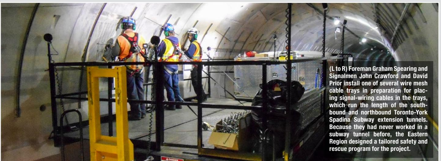
(L to R) Foreman Graham Spearing and Signalmen John Crawford and David Prior install one of several wire mesh cable trays in preparation for placing signal-wiring cables in the trays, which run the length of the southbound and northbound Toronto-York Spadina Subway extension tunnels. Because they had never worked in a subway tunnel before, the Eastern Region designed a tailored safety and rescue program for the project.
