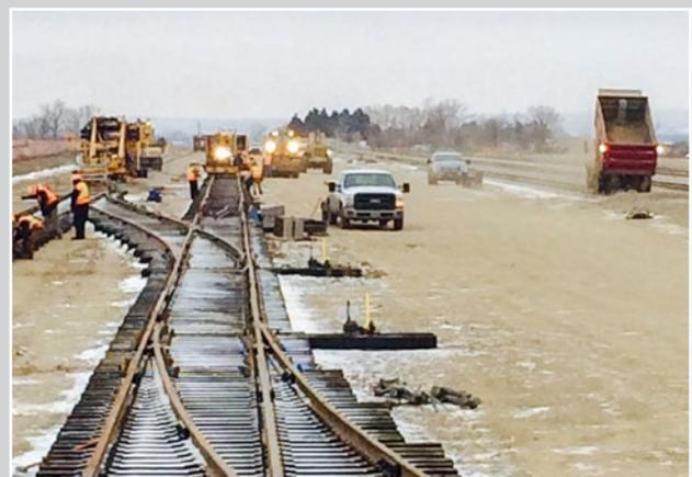
Crews construct track and turnouts, spread ballast and tamp at NorthStar Transloading terminal in East Fairview, ND.
