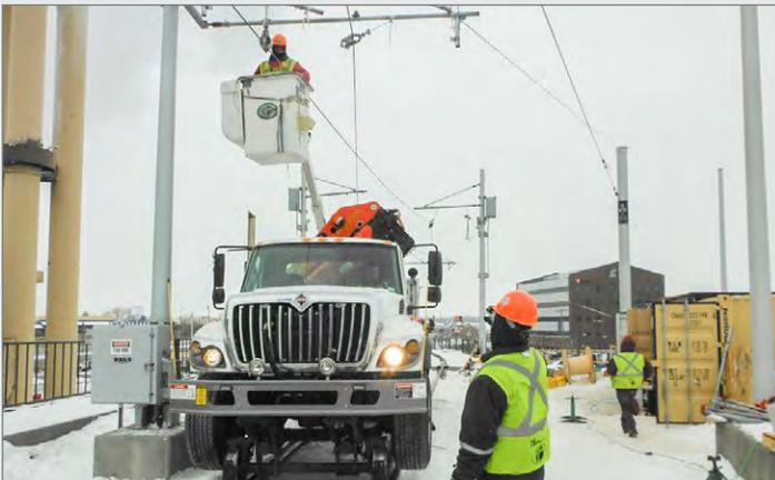
Delays in turning over work have caused L.K. Comstock National Transit crews to work during the harsh Minnesota winter to install the overhead catenary system (OCS) for The Interchange project. Record cold and snow – about 50 inches this winter – have challenged crews working to wrap up work by March 8, when the new OCS ties into the existing system.
