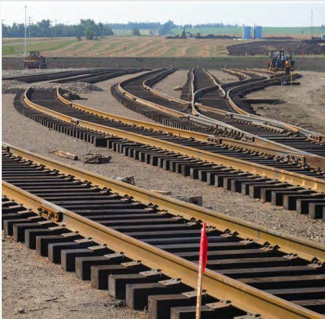
PNR RailWorks first constructed 18 tracks to create a rail car storage area at Canexus' Bruderheim Terminal. This area provides capacity for 109 tanker cars, which contain chlor-alkali used in horizontal drilling and fracturing operations in Western Canada.
