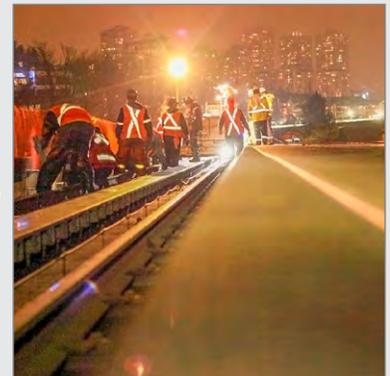
**PNR RailWorks crews work at night on an elevated structure to change out power rail components on the Expo Line in Greater Vancouver, British Columbia.**
