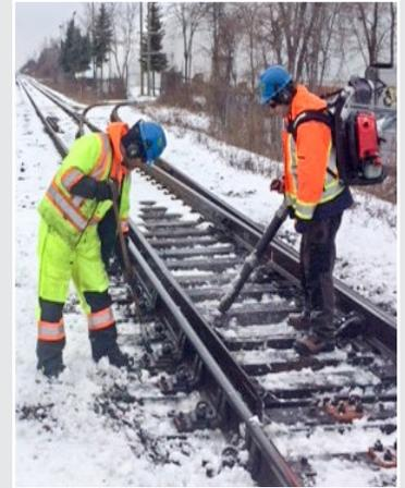
Kyle Charette, right, uses a backpack blower to remove snow from switch points and rods, while Track Maintainer Mike Tenant is using a broom with a scraper to remove any excess ice from the base of the rail to allow the switch point to close correctly. Kyle and Mike are part of PNR RailWorks' GO Transit Maintenance Division.
