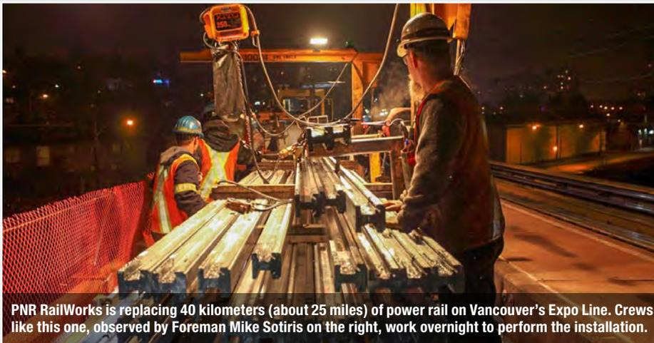
PNR RailWorks is replacing 40 kilometers (about 25 miles) of power rail on Vancouver's Expo Line. Crews like this one, observed by Foreman Mike Sotiris on the right, work overnight to perform the installation.
