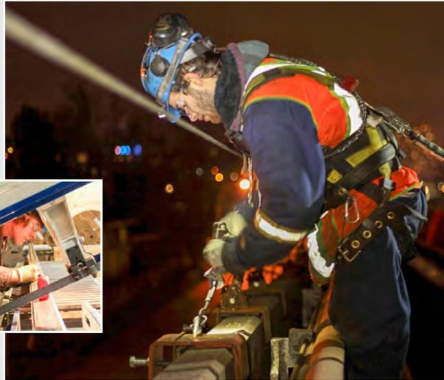
**Machine Operator Jeremy Naman, above, erects a stanchion post for a pivoting guard rail on the Expo Line guideway. Inset: Trackman Bill Jamieson marks power rail before cutting it to size for transportation and installation.**
