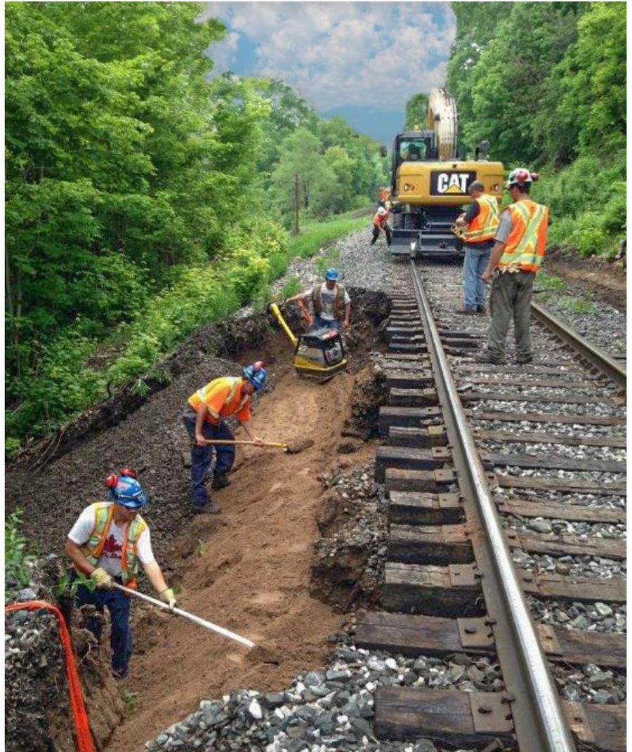
PNR RailWorks crew members compact gravel to protect the fiber-optic cable prior to restoring the rail bed after a washout at mile post 10.2 on GO Transit's Bala Subdivision.
