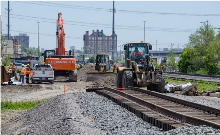
Work under way on GO Transit's Georgetown South Corridor
