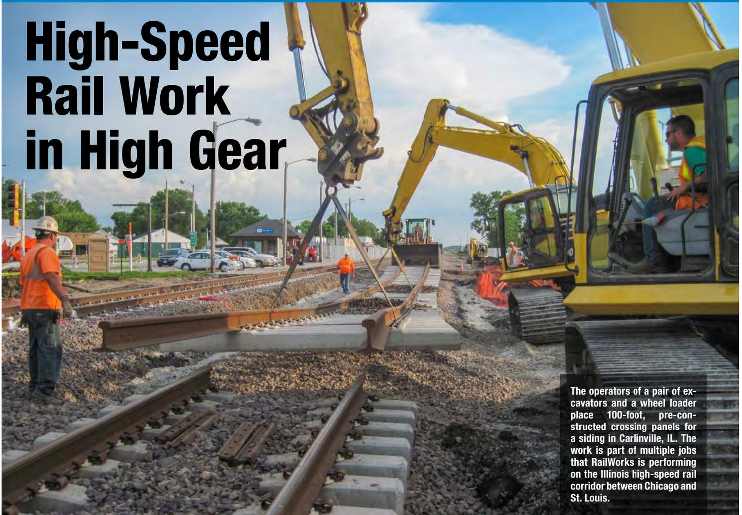
The operators of a pair of excavators and a wheel loader place 100-foot, pre-constructed crossing panels for a siding in Carlinville, IL. The work is part of multiple jobs that RailWorks is performing on the Illinois high-speed rail corridor between Chicago and St. Louis.
