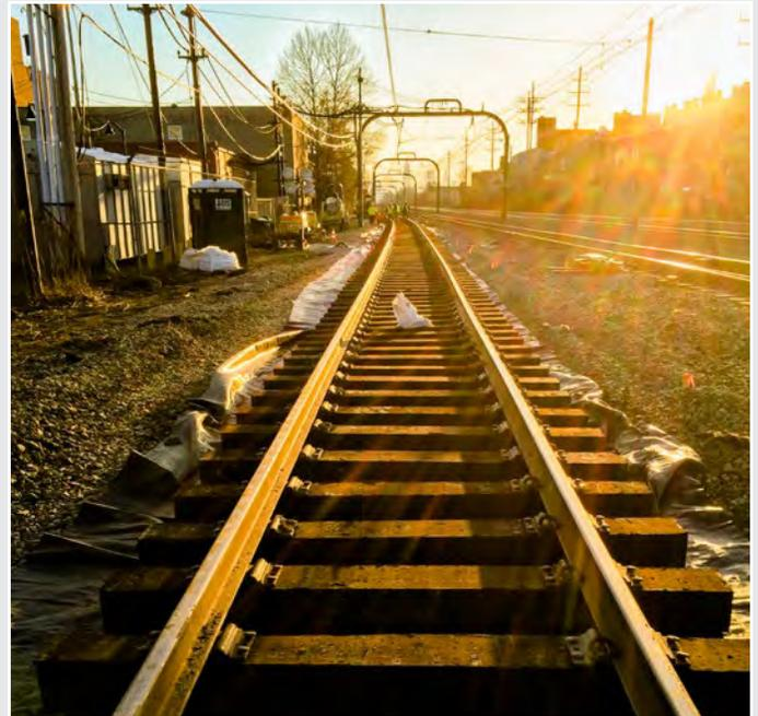
A view east from the 117th Street Station platform highlights a key project challenge: reconstructing the track around both overhead and underground cables and installing drainage between a traction power duct bank and a signal duct bank. Every wire for a 2-mile segment of the track returned back to these two structures.
