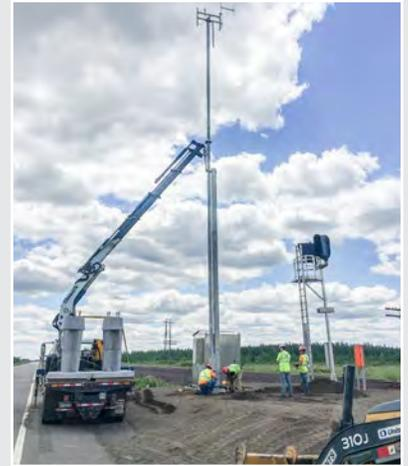
Working just south of Virginia, MN., on CN's Rainy & Missabe Subdivision, RailWorks Signals & Communications Foreman Craig "Bubba" Knowles and his crew install and erect an antenna on a wayside tower. This equipment is part of a Positive Train Control (PTC) system, which is federally mandated on railroad main lines with regularly scheduled intercity passenger or commuter rail services or that are the route for any poisonous-inhalation-hazardous (PIH) materials.
