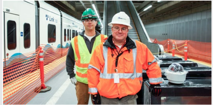
Project Manager Juan Estrada, foreground, and Foreman Patrick Ritter stand alongside a Sound Transit light rail train during the final testing and commissioning of the U Link communications system.
