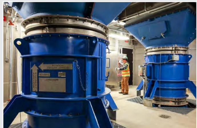
**Foreman Patrick Ritter works in the Capitol Hill Station fan room to check the wiring of the control panel for fans and dampers. The large blue fans are part of the Emergency Ventilation System and control exhaust air flow in the train tunnel.**
