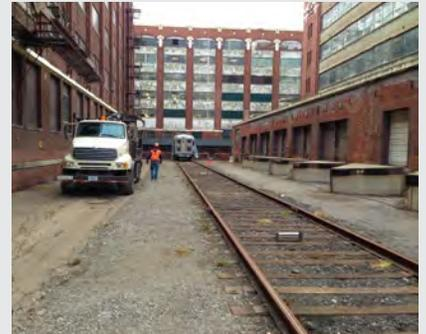
"We were able to construct each of the sets in two day's time," says Dan. "The track through the parking lot was filled, leveled and hand tamped using asphalt grindings to create a worn and aged appearance. The elevated track set utilized a good portion of relay materials from stock that will again be re-claimed as well as materials deemed scrap from the other recent projects."
