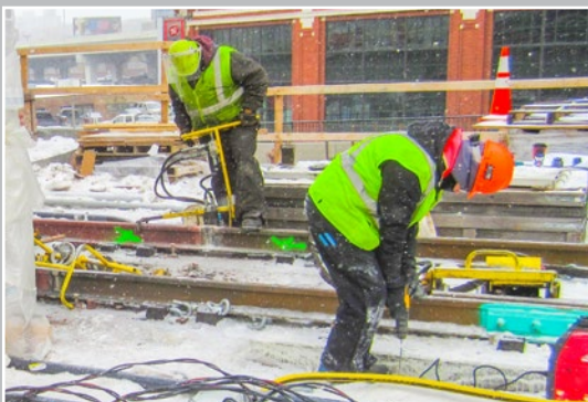
A RailWorks Track Services employee (at left) grinds a weld on the rail while an L.K. Comstock National Transit electrician drills holes in the guideway to install anchors for a train-to-wayside-communication (TWC) loop. Crews on The Interchange often worked in frigid temperatures, as they did on this January day. In the photo at right, RailWorks' work is on display at the south end of Target Field Station. Junction boxes, switch machines and conduits for switch heater cables can be seen in the foreground. A double crossover is visible in the background.
