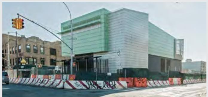
NY Transit crews have performed the civil and electrical work for the new, two-story relay room, which will replace a smaller, outdated relay room dating back to the 1950s. The new structure features the latest communications, fiber optic network, security controls, inergen fire protection and associated HVAC equipment systems, as well as new communications-based train control (CBTC) signal system technology.
