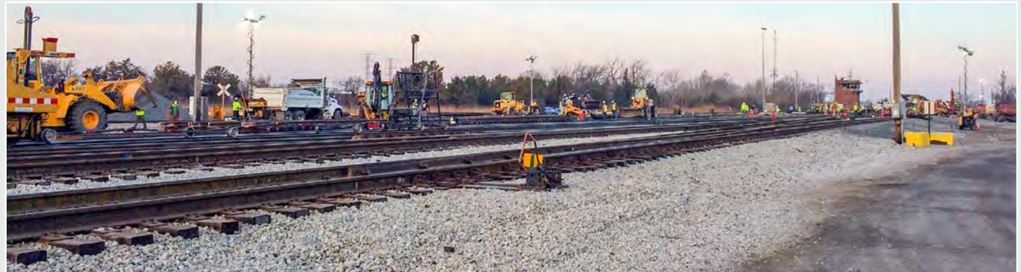
RailWorks and other contractors performed a range of work during the 32-hour outage Oct. 27 and 28 at CN’s Kirk Yard in Gary, IN, including replacing turnouts and signals, making thermite welds and surfacing track. Shown here at the west entrance, contractors had to carefully coordinate personnel and equipment through the yard’s only access point.
