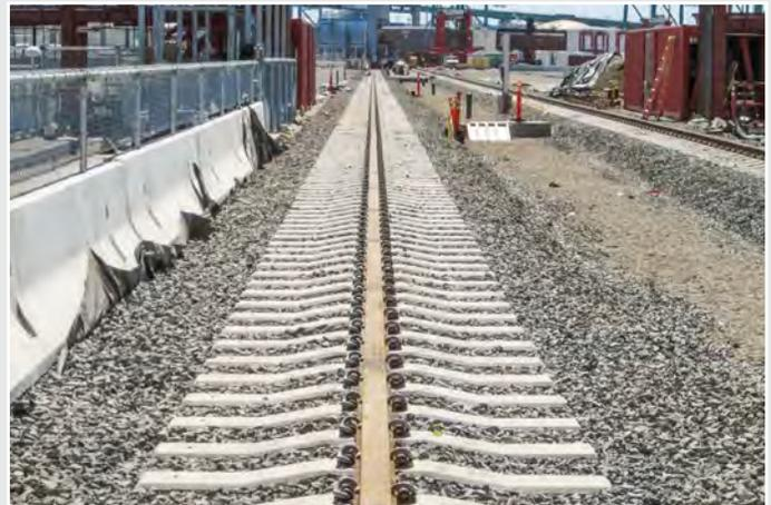
At left, a crew at the Port of Los Angeles threads continuous welded crane rail at a TraPac terminal during upgrades there. RailWorks installed six crane rail tracks like the one on the right, with a tolerance limit of 2mm, at TraPac's new, fully automated cargo container handling facility.
