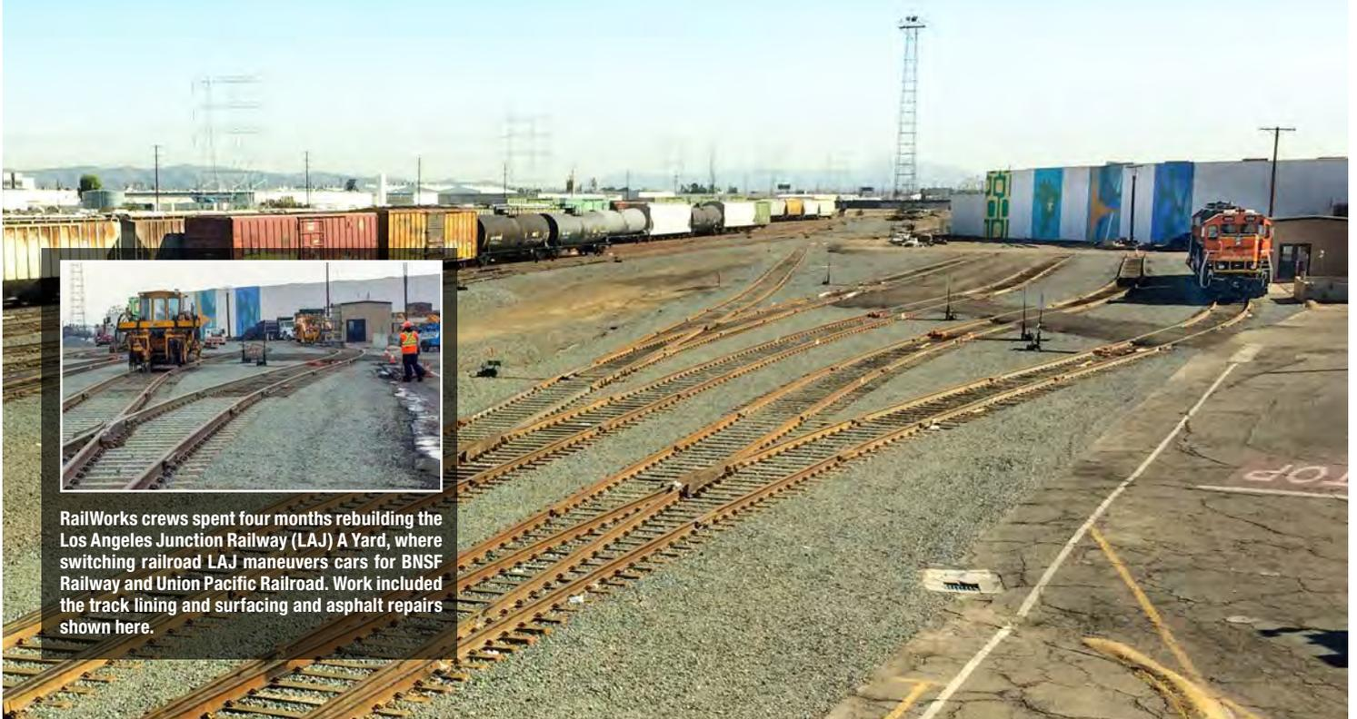
RailWorks crews spent four months rebuilding the Los Angeles Junction Railway (LAJ) A Yard, where switching railroad LAJ maneuvers cars for BNSF Railway and Union Pacific Railroad. Work included the track lining and surfacing and asphalt repairs shown here.
