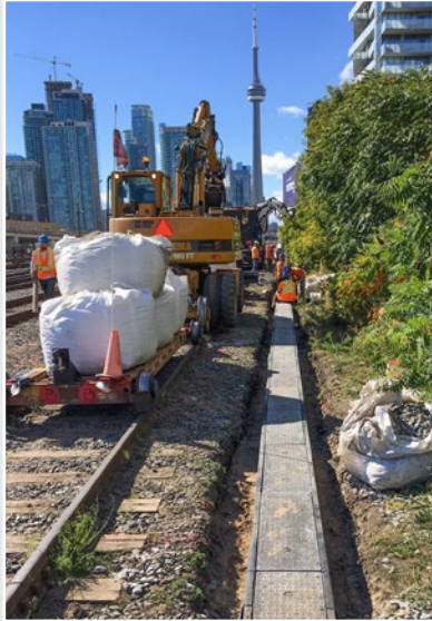
Working west toward Union Station in the shadow of the CN Tower in Toronto, ON, PNR RailWorks signalmen installed troughing into an excavated trench.
