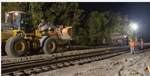
Removing the old track panel in preparation to install a #20 turnout
