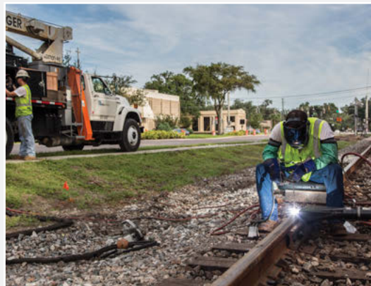
Welding rail at the new crossing installations
