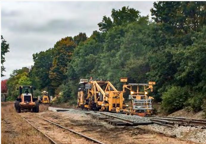
This turnout in Willimantic, CT, is one of nine that RailWorks is installing on the New England Central Railroad.
