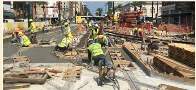
Working in extreme heat and high humidity, crews completed constructing the track for the half grand union in New Orleans just after it was encased in concrete. Workers constructed the special trackwork featuring six switches and a crossing diamond at the intersection of Canal and North Rampart streets, where the existing and new streetcar extension connect.
