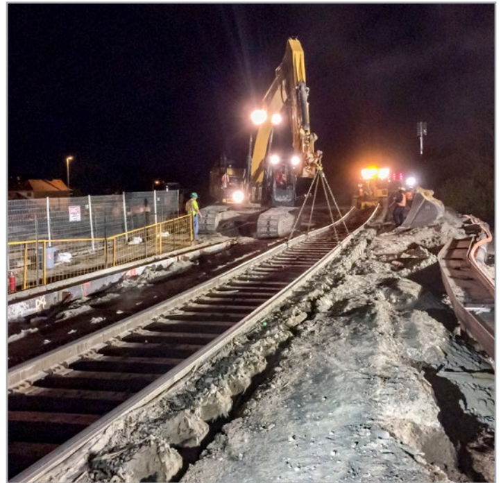
A track crew removed and reinstalled 90-foot track panels during the project.
